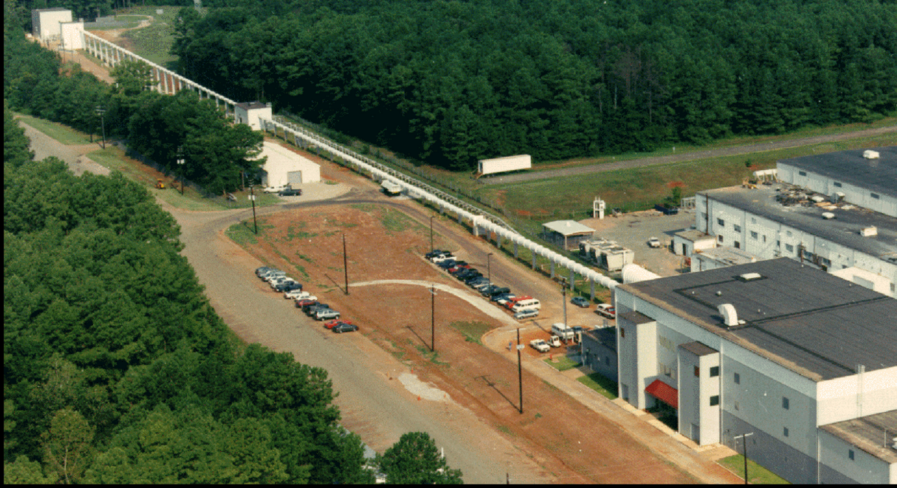
Marshall Space Flight Center (MSFC) X-ray Calibration Facility with its 520m X-ray Tube
